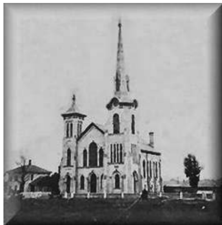
The new 1873 "Cathedral Church."
